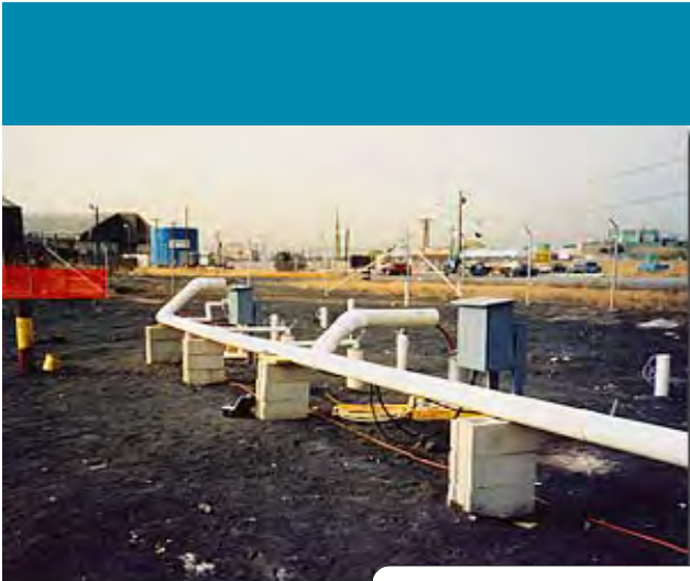
Soil Vapor Extraction / Air Sparging
